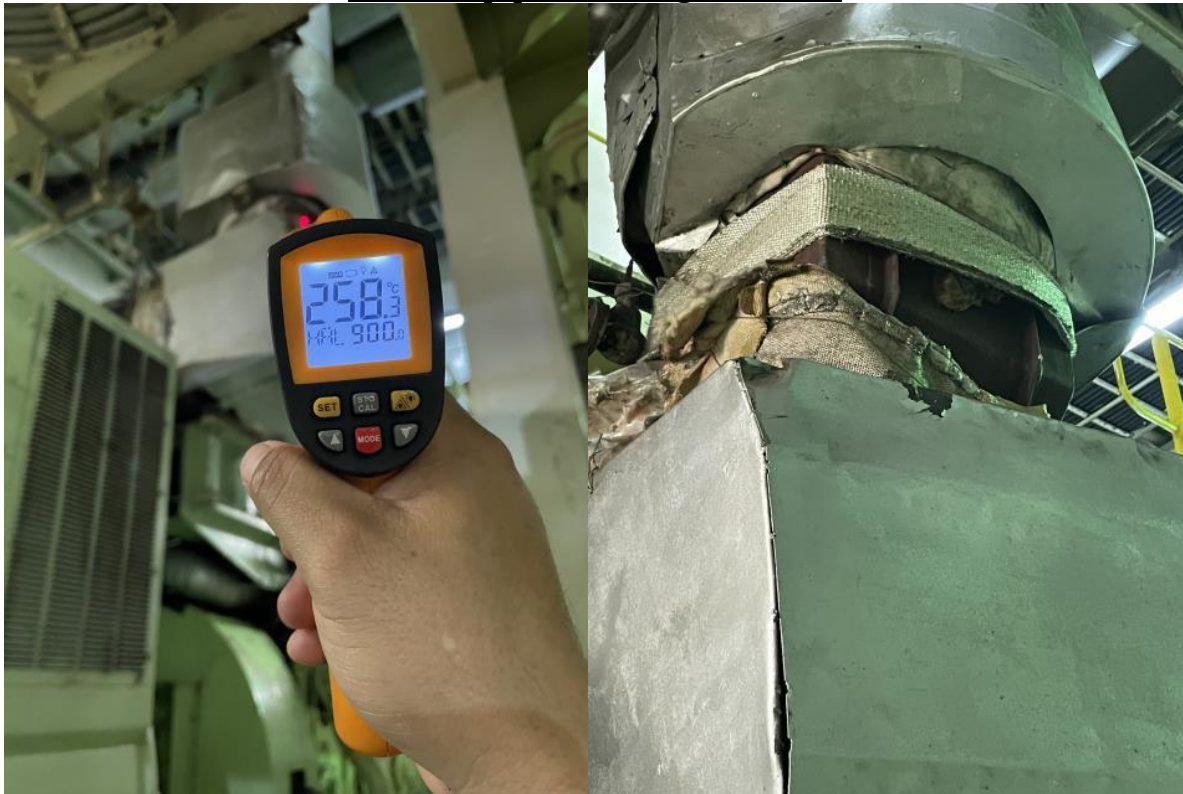
Pictures of other deficiency: Section of insulation missing on the turbocharger exhaust pipe of all 4 generators
