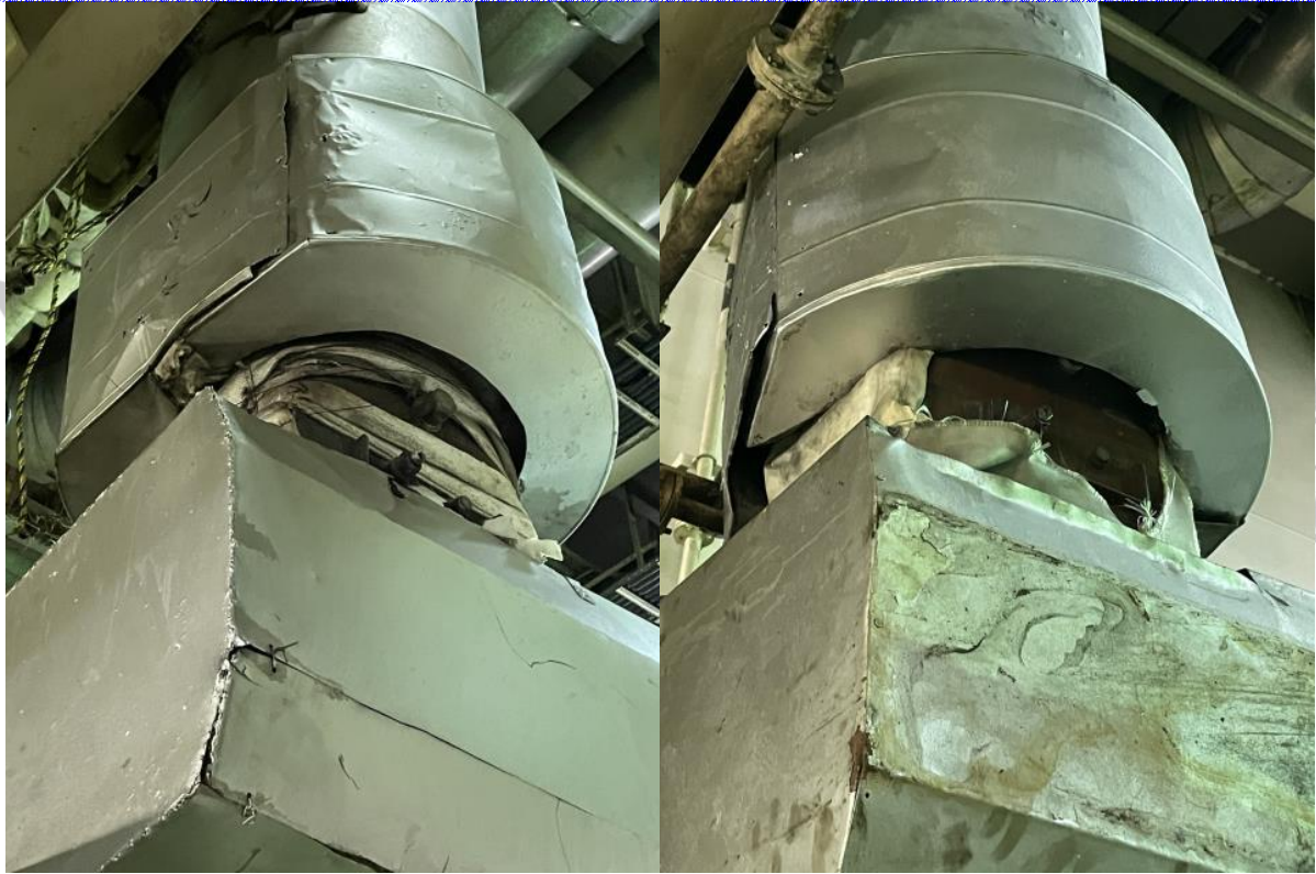
Picture of other deficiency: Fresh water generator outlet pipe temporarily repaired with doubler
