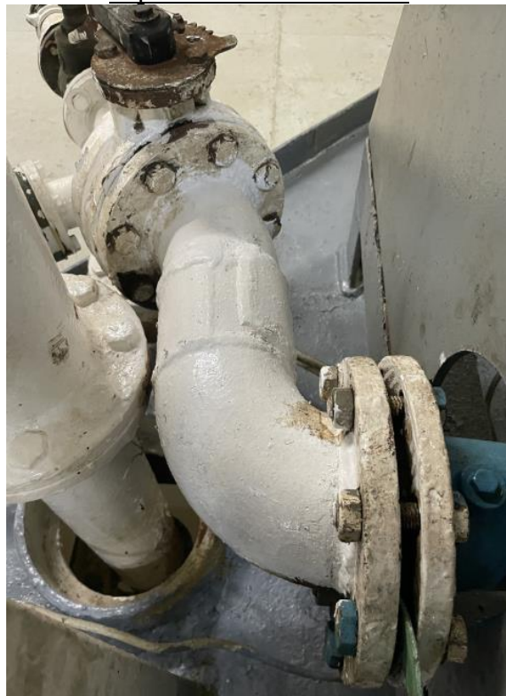
Picture of other deficiency: Fresh water generator outlet pipe temporarily repaired with doubler
