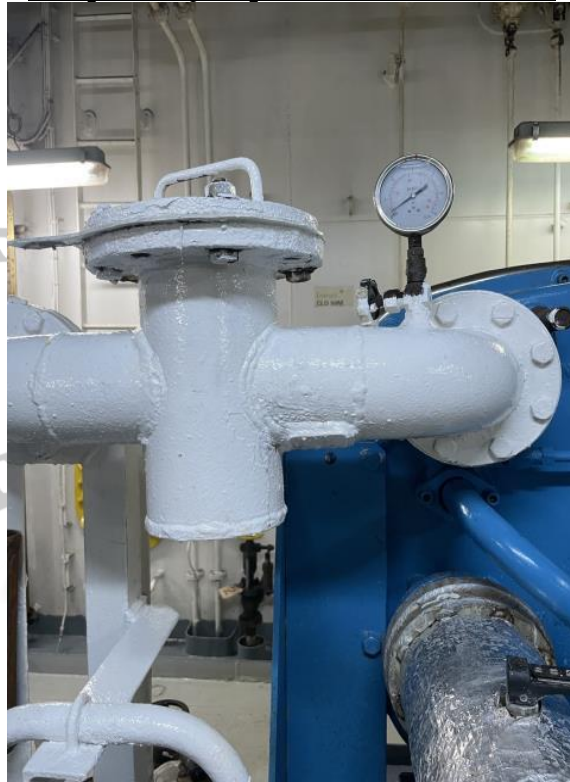
Picture of other deficiency: Main engine jacket water cooler seawater outlet pipe temporarily repaired with doubler
