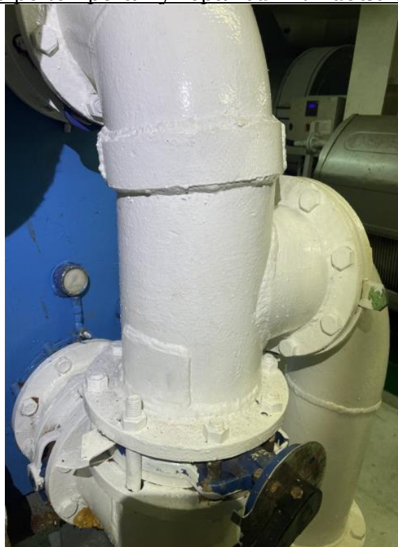
Picture of other deficiency: Main engine jacket water cooler seawater outlet pipe temporarily repaired with doubler
